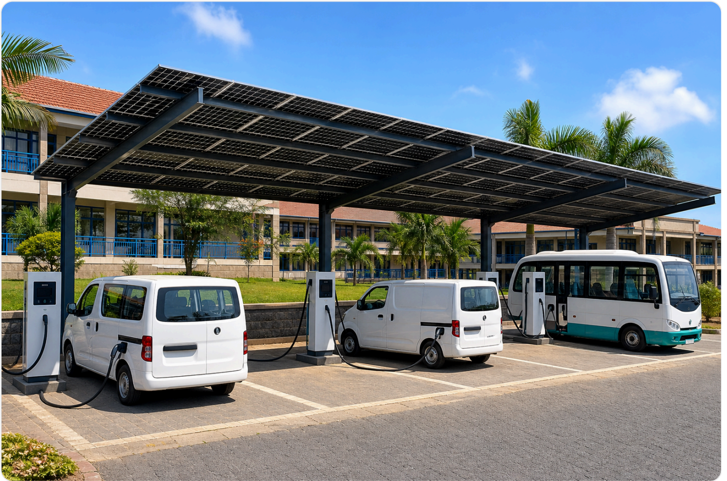
Figure 7 — Private in-house / campus station: multi-pedestal solar canopy site.
