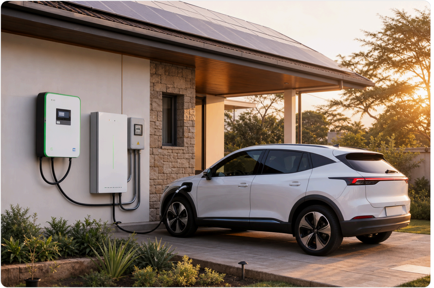
Figure 8 — Private house hybrid install: wall charger, rooftop solar, home storage.
